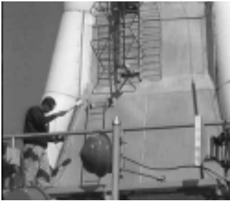
Some sites contain both wireless and broadcast systems.
